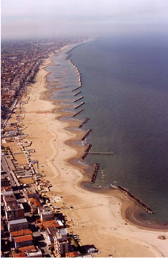
Fig. 1. Coastal defence structures along the Italian coasts of the north Adriatic sea
